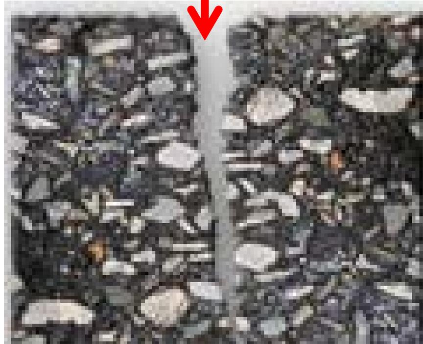
Rout the crack keeping the cutter centered over the crack
